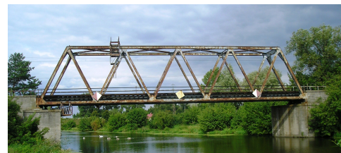
Figure 1. Investigated railway truss bridge in Nieporęt.
