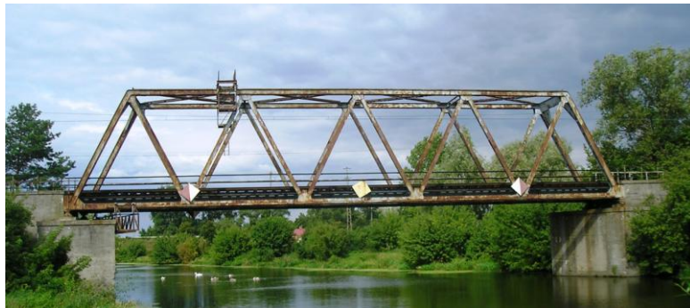
Fig. 1 Investigated railway truss bridge in Nieporet
