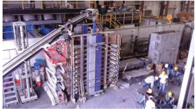
Fig. 2: Construction of full-scale mockup (left), previously constructed mockup (back, right) and specimen casting for materials testing during recent investigation of delamination of the concrete containment structure in Florida's Crystal River Nuclear Power Plant, led by Georgia Institute of Technology, with funding from the Electrical Power Research Institute (EPRI) (photo courtesy of Kimberly E. Kurtis)
