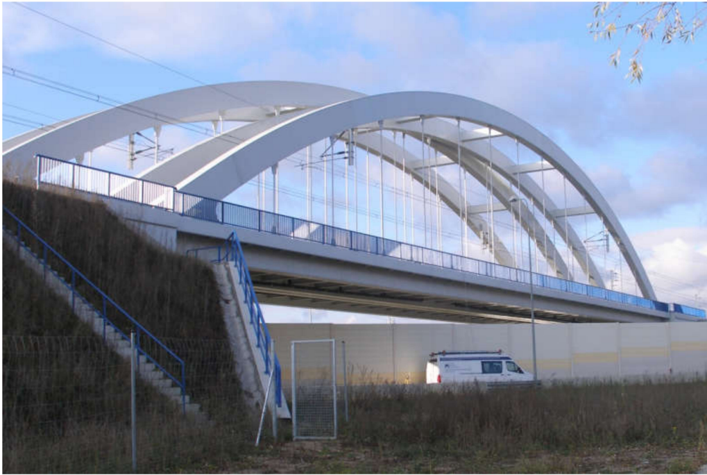
Figure 3. View of the tested bridge.
