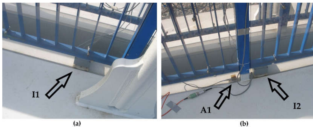
Figure 5. View of inclinometers and accelerometer location: (a) Inclinometer I1 location; (b) accelerometer A1, and inclinometer I2 location.
