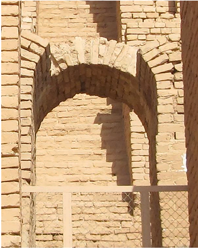
Fig. 1. A semi-circular arch made of clay brick and gypsum mortar, Choga Zambil, Susa, 1250 BCE.
